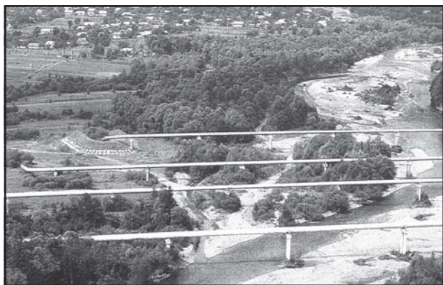
Fig. 8.17: Pipelines transporting natural gas in Ukraine
